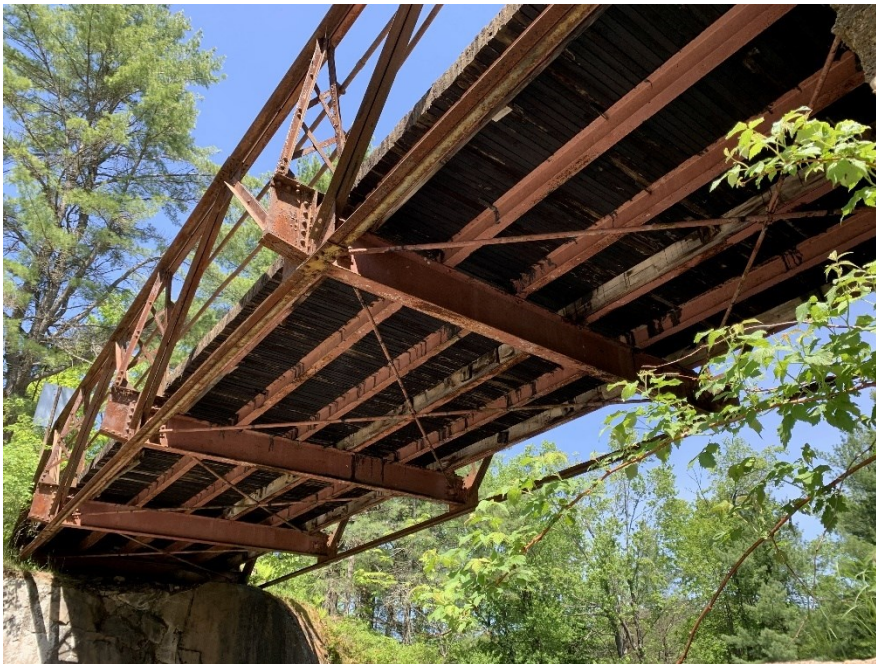
Plate 8: Underside of the western Warren truss span, stringers and floor beams visible.
