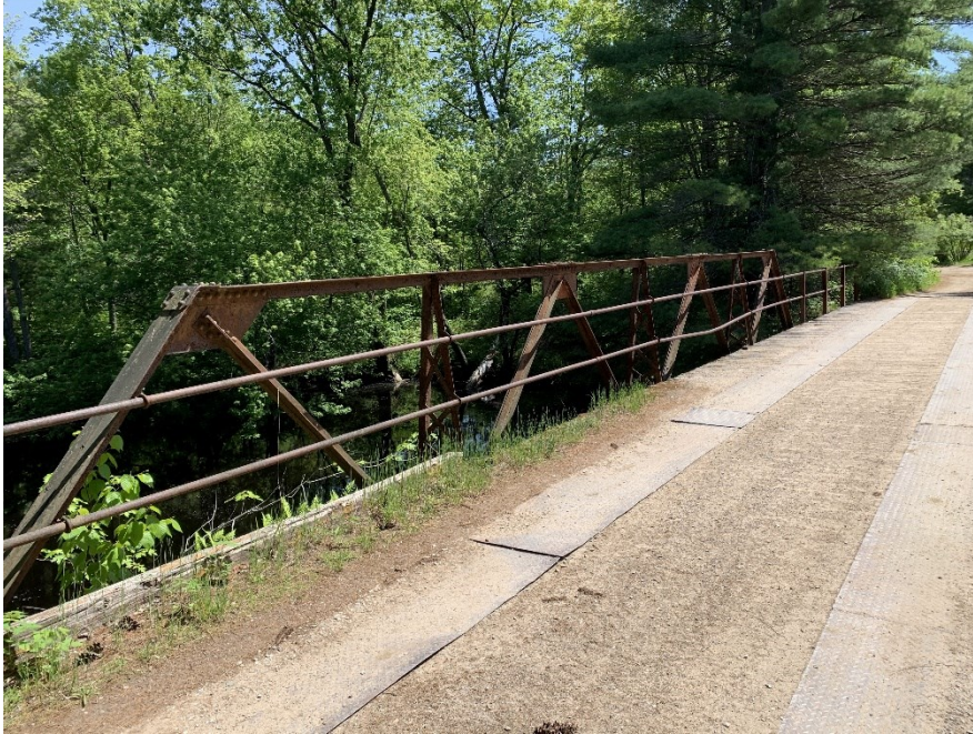
Plate 5: View of the north truss and double steel rail-barrier and bridge deck.
