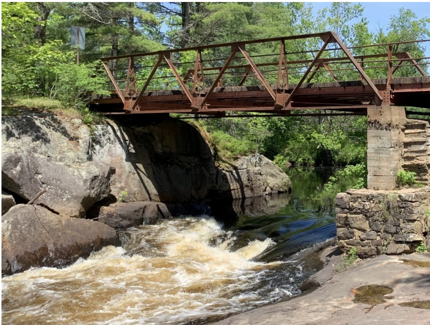
Plate 10: Natural rock that makes up the western abutment.
