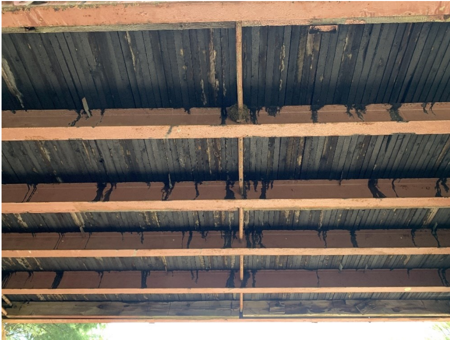
Plate 9: Underside of the eastern deck girder span, rolled steel I-beam stringers visible.
