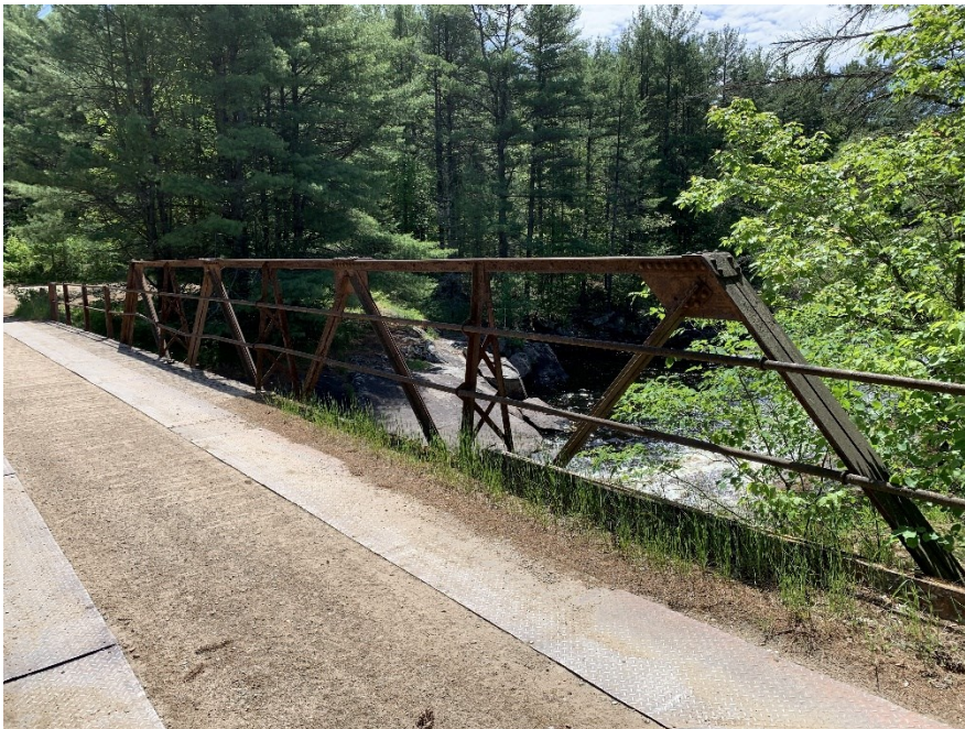
Plate 6: View of the south truss and double steel rail-barrier and bridge deck.
