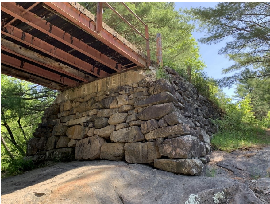
Plate 11: Dry fit stone of the eastern abutment.
