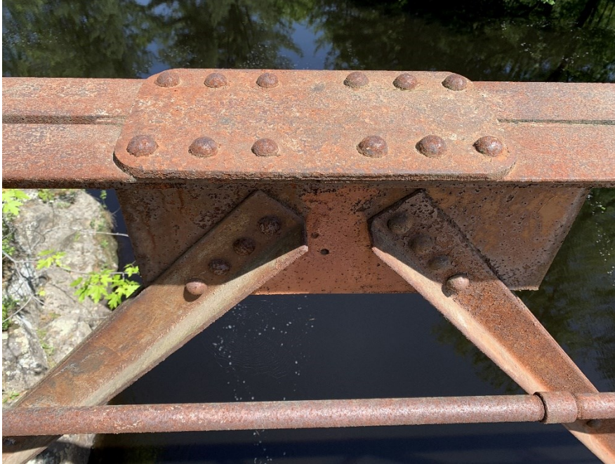
Plate 7: Close-up of the riveted steel connections of the truss. The steel pipe railing system is visible below.
