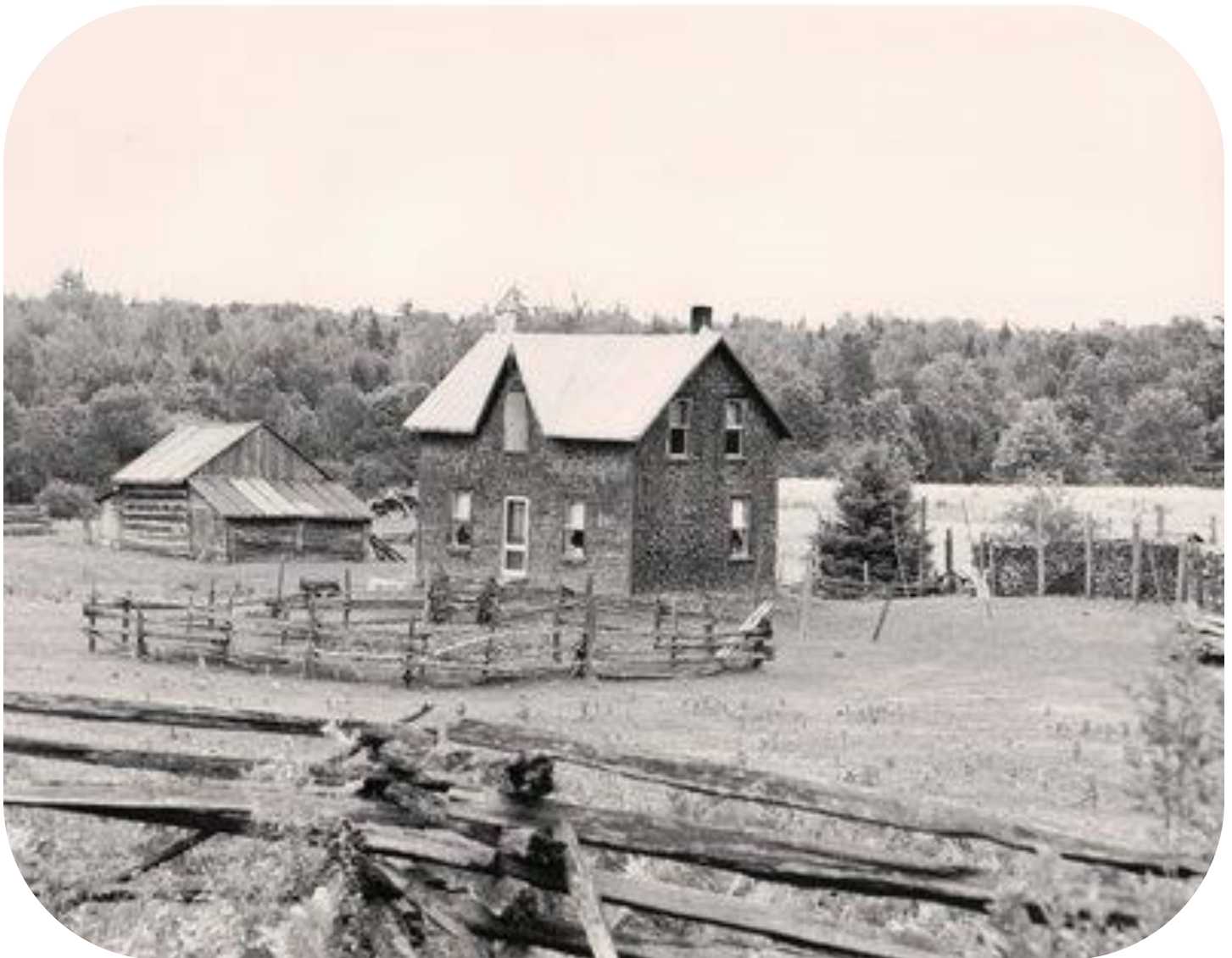
Farmhouse, Somerville Township, built mid to late nineteenth century
