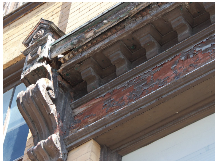
This decorative woodwork requires repair and re-painting to ensure that it does not deteriorate.
