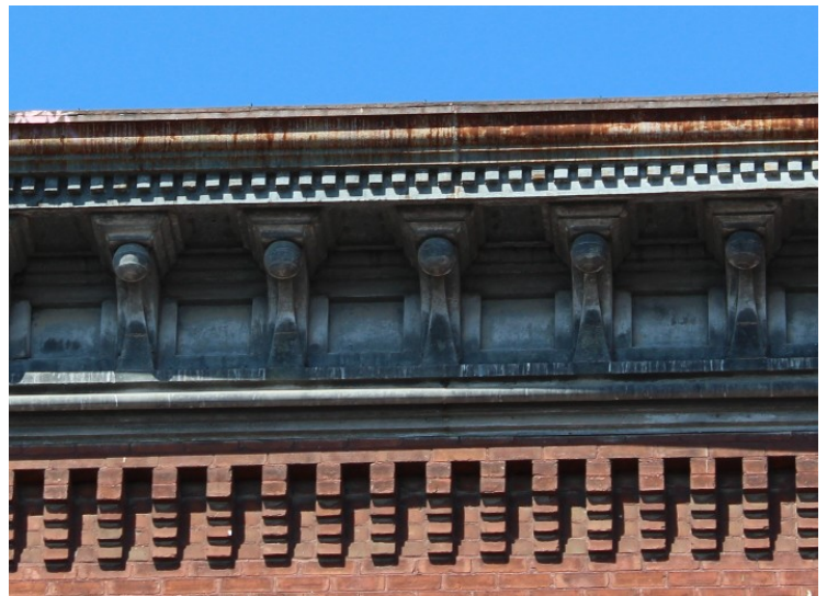
Metal elements such as cornices should be kept rust free and repainted as necessary to avoid deterioration.
