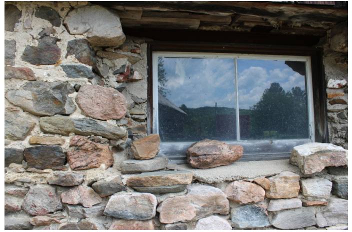
The foundation around this window requires repointing and repair to replace the dislodged stones
