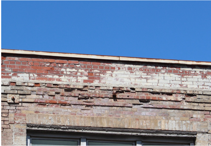
This masonry is badly deteriorated and requires replacement bricks and repointing
