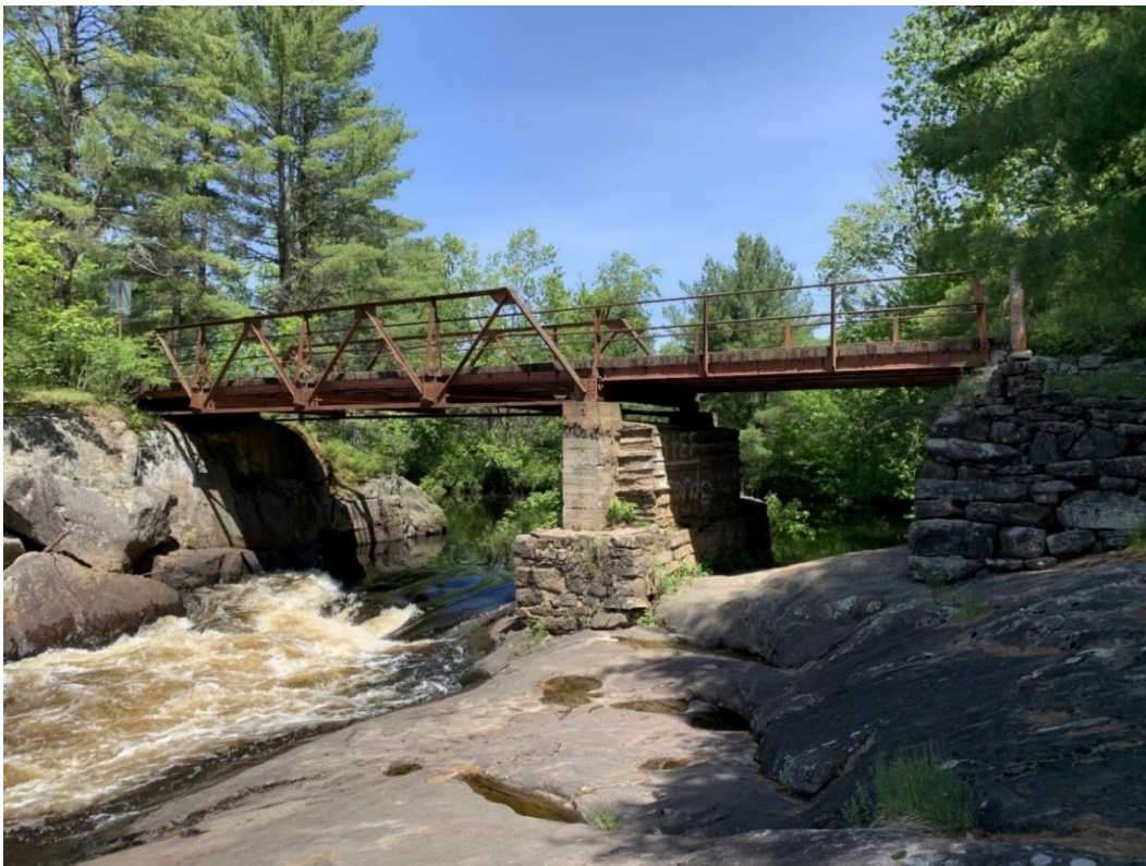
Figure 3: South elevation of the subject bridge showing the half-through Warren truss main span on the left and deck girder approach span on the right (ASI 2020)
