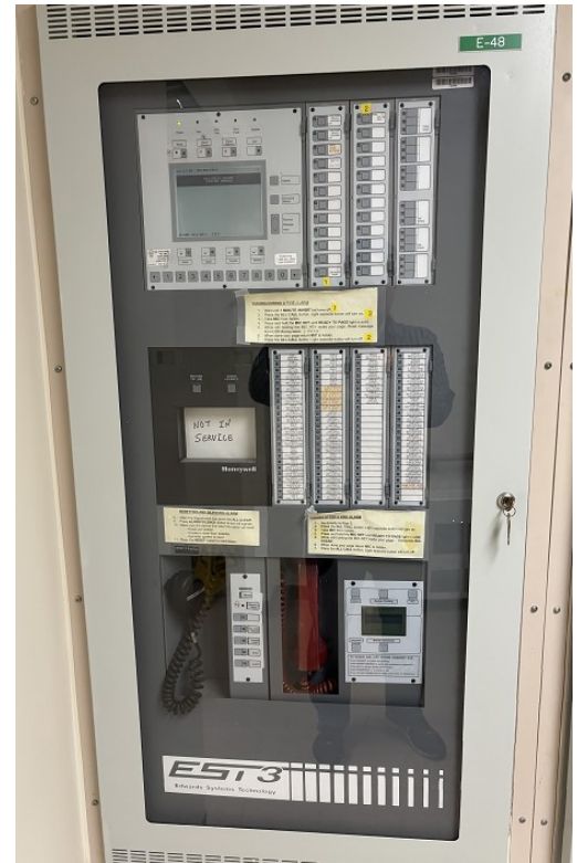
Fire Annunciator Panel Main Fire Panel
