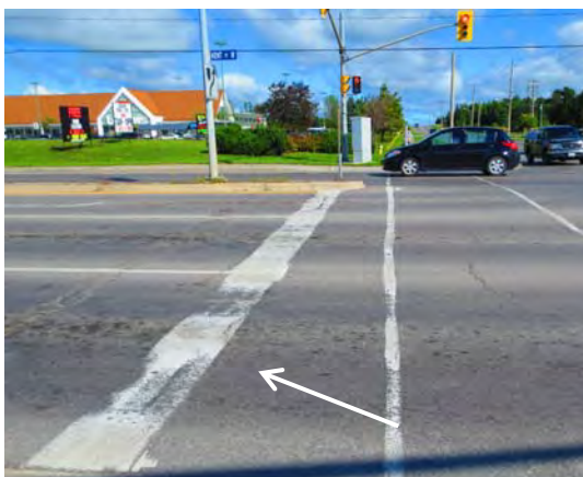
Exhibit E: Faded pavement marking at St. Joseph / Kent (west leg)
