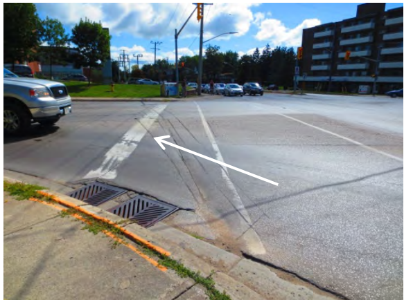
Exhibit D: Faded stop bar and cracking in pavement at Angeline / Kent Street (north leg)
