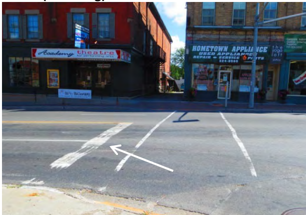
Exhibit C: Faded Stop bar at Lindsay / Kent Street (north leg)
