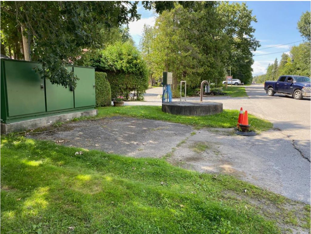
Front St SPS Wet Well Chamber and Control Panels (above ground equipment)
