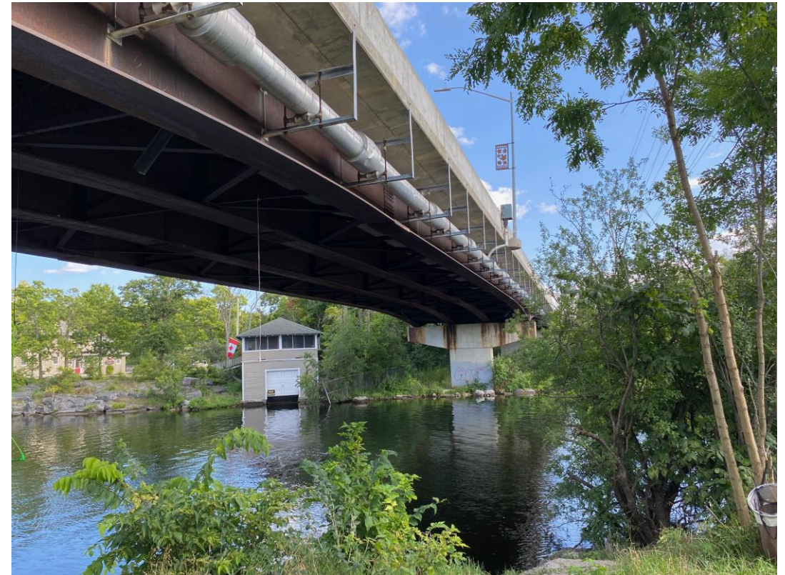
300mm diameter Forcemain on East St. Bridge to WWTP
