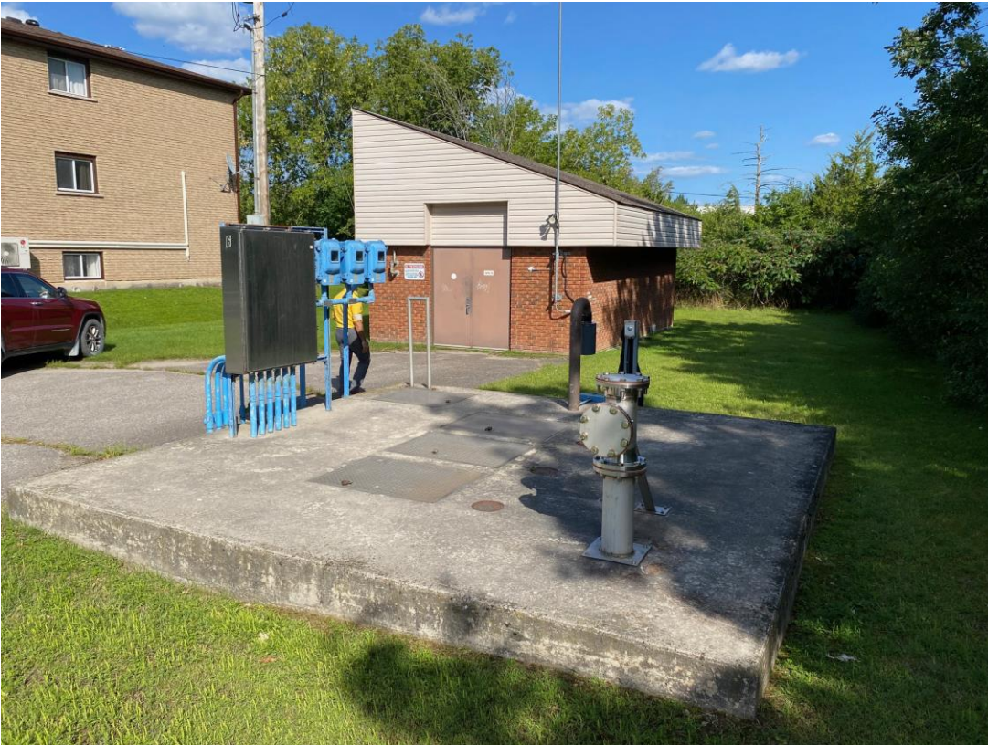
SPS Wet Well Chamber, Control Panels and Emergency Power Generator Building
