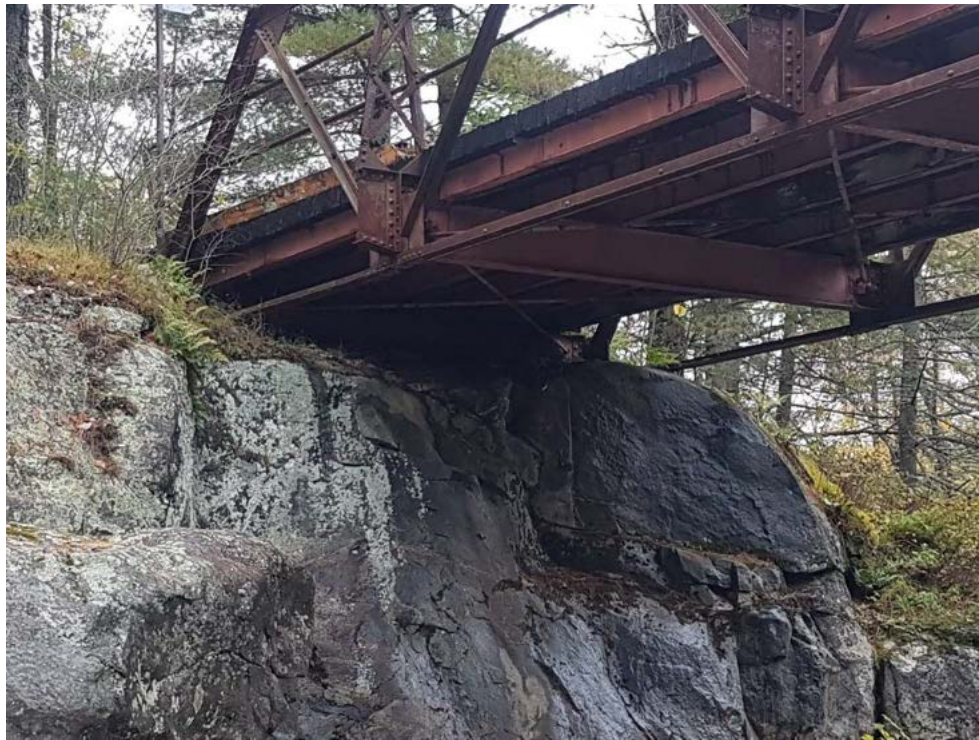
Photo 7 – West End Bearing on Bedrock
