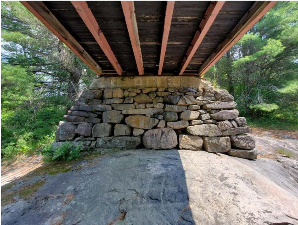
Photo 5 – East Stacked Stone Wall Abutment with Concrete Top
