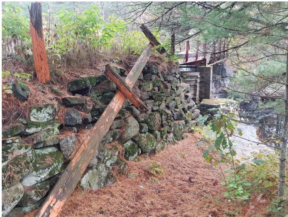
Photo 8 – Broken Wooden Approach Rail, Northeast Quadrant
